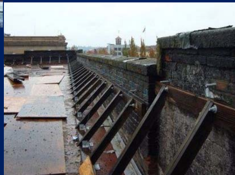
Bracing of URM parapets keeps them from toppling to the sidewalk below
