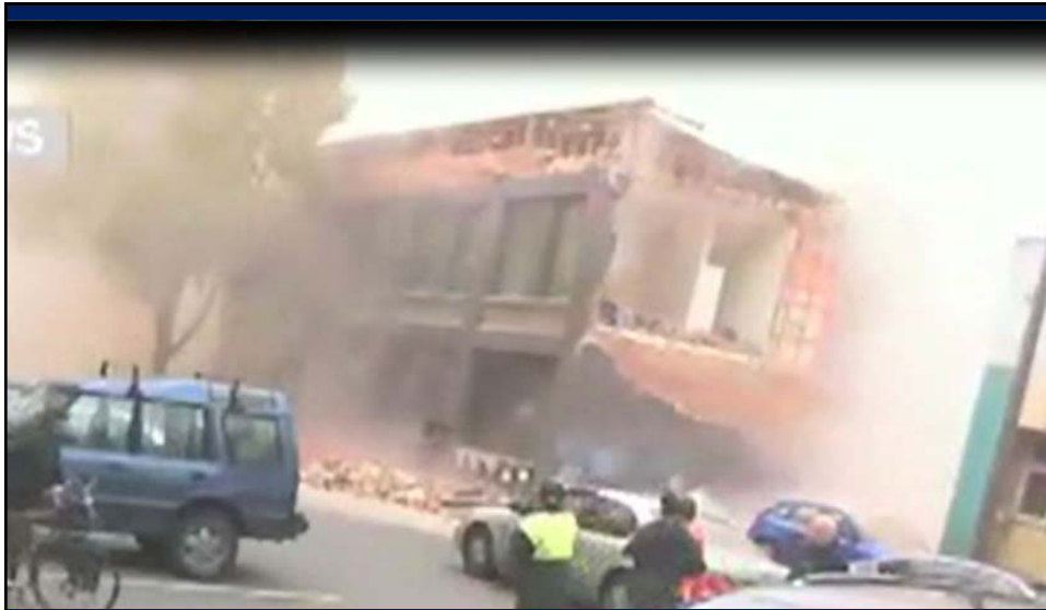
Damaged URMB – major failure of right facing wall exposing rooms and Failure of the upper part of the left facing wall. Debris surrounds building.
