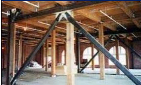
Interior cross bracing helps prevent building collapse
