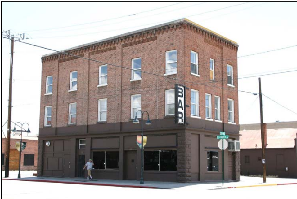
Three story URBMB with some earthquake cracks; occupancy is variable
